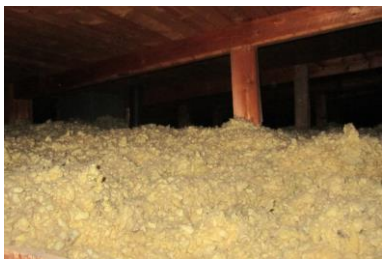
Figur 2: Takisolering 400-500mm tjock
